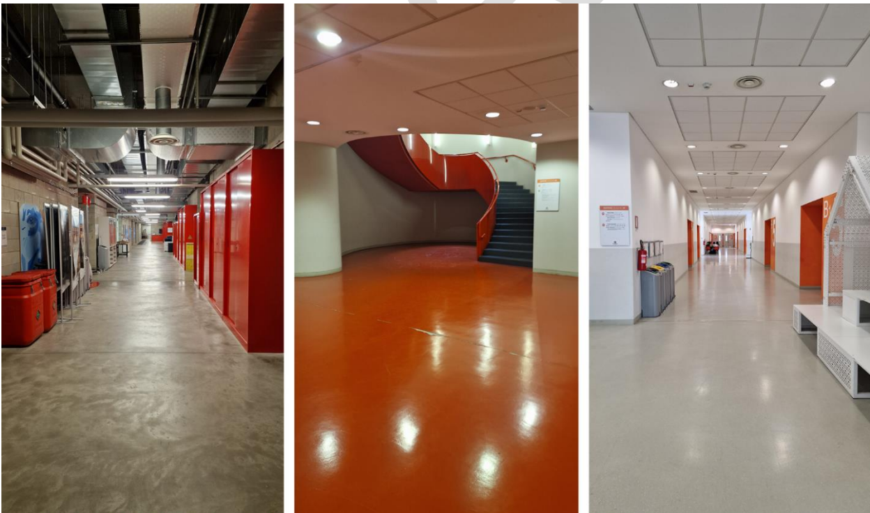
Figure 38: Internal view of the first floor of building 9. On the left side is shown the distributive corridor in the underground floor. In the middle it's show the main stair. On the right side the distributive corridor, common in all the floors above ground.
