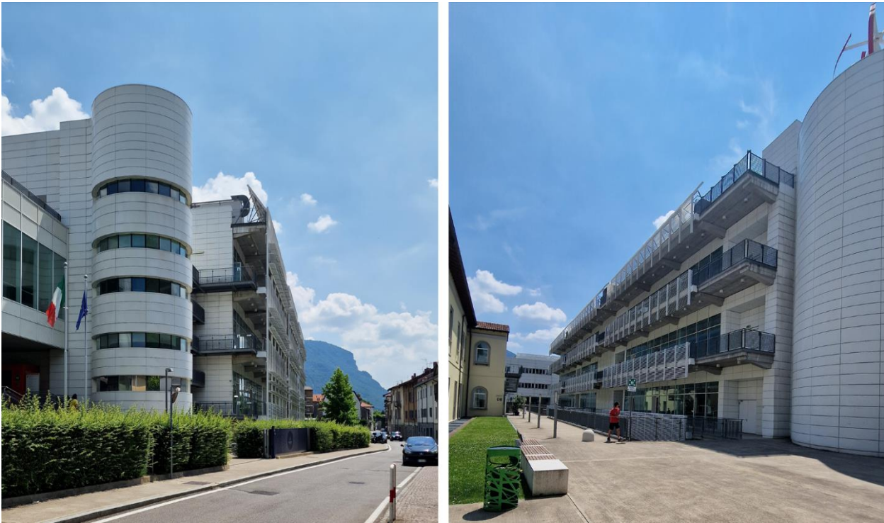
Figure 37: External view of building 9. On the left side the west façade view, on the right side the east façade view.
