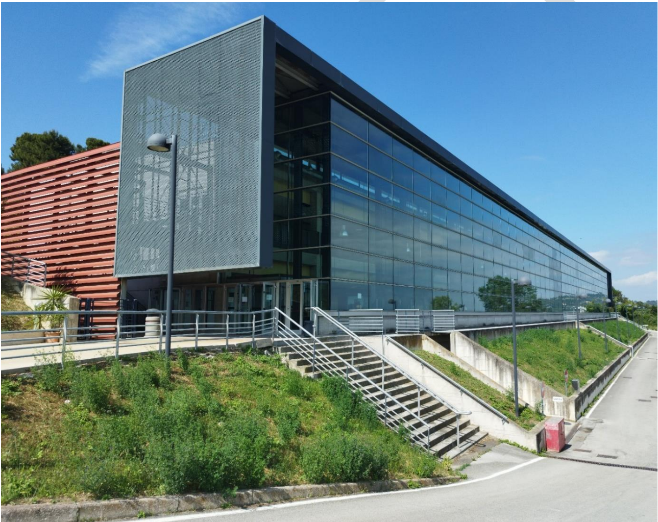
Figure 29: BAS north façade view.
