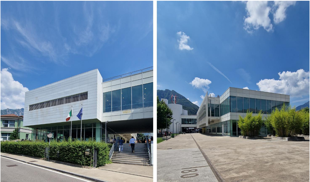
Figure 35: External view of building 10. On the left side the west façade view, on the right side the east façade view.
