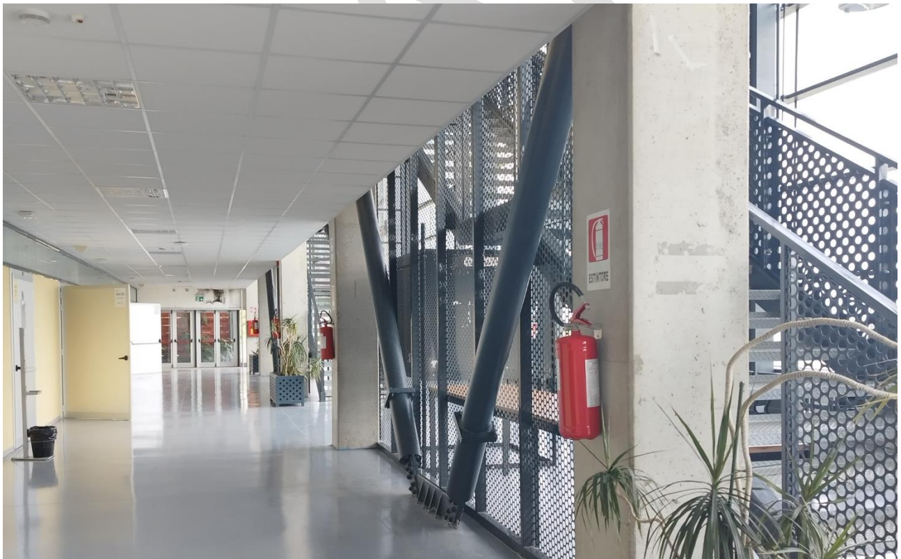
Figure 31: Detail of a dissipative brace.
